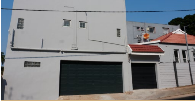
Roofing & Waterproofing: Comprehensive roof refurbishment and specialised waterproofing treatment at 23 St Thomas, resolving historic leak vulnerabilities with reinforced membrane sealing and precision joint flashing to guarantee complete weather protection.
