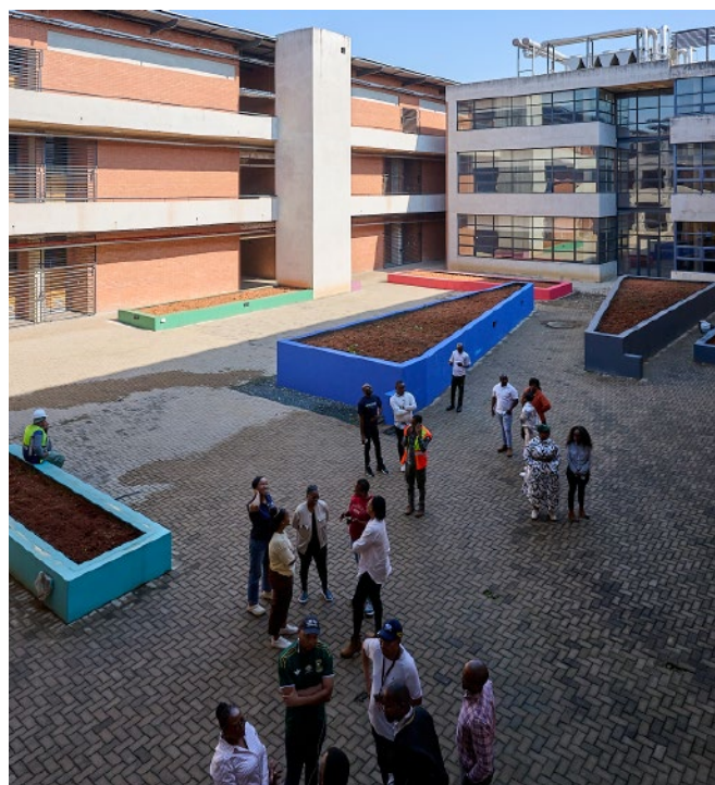
Indumiso Campus: Engineering Building under construction
