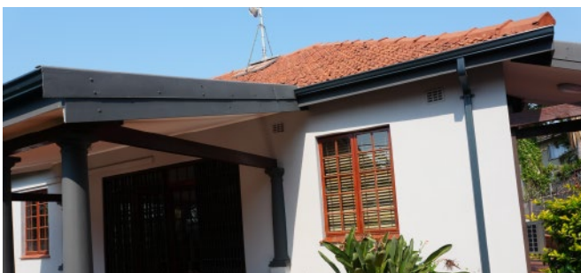
23 St Thomas: (Exterior Façade & Covered Veranda Restoration) Completion of structural and aesthetic upgrades to the front elevation at 23 St Thomas, showcasing freshly treated charcoal-painted support pillars, revitalised exterior masonry, and restored roof eaves with integrated rainwater gutters. The spacious tiled patio and curated garden bedding enhance the property's architectural character while delivering a durable, high-standard exterior finish.
