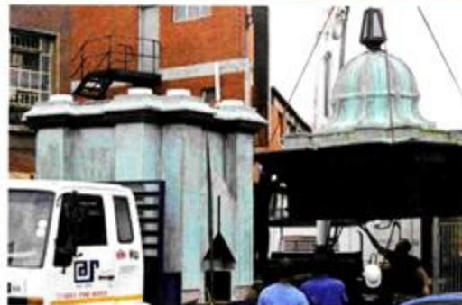
The Bell Tower was assembled into various sections and delivered to the site where it was hoisted by crane and attached to a steel structure by Mouldform's fixing crew
